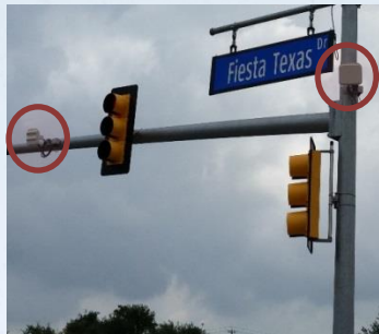
Steel Mast Arms & Vehicle Detection
